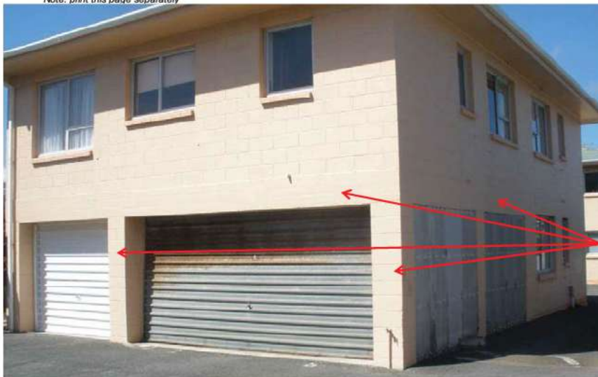
West-South Wall showing large penetrations at ground level
