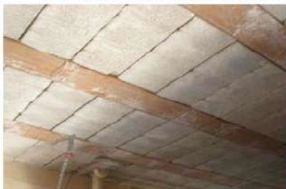
Exposed Brick Beam and Hollow Block at Garage Area Upper Floor
