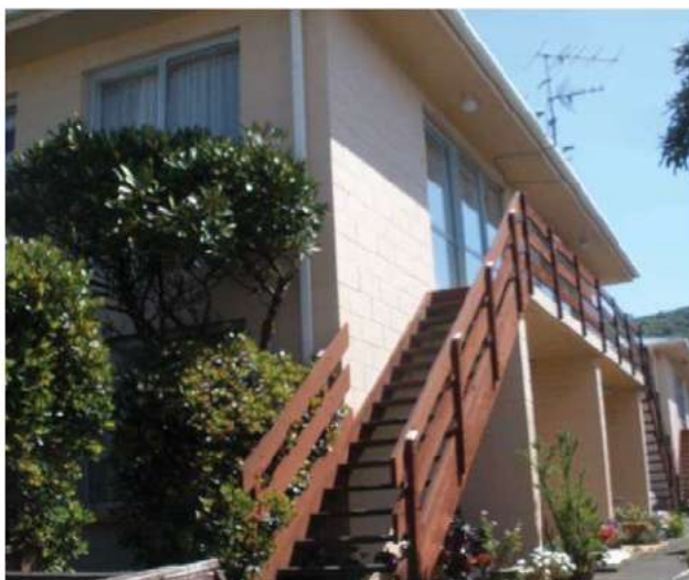
North wall showing large penetrations and good width of remaining wall
