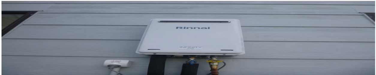
The continuous hot water system in good condition but not operational at the time of inspection
