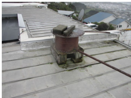
header tank on roof
