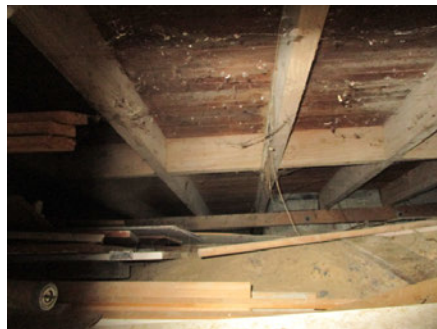
underfloor not insulated in area sighted
